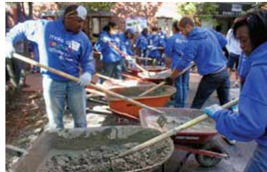
Volunteers mixed more than 13,000 pounds of cement to secure the playground.
