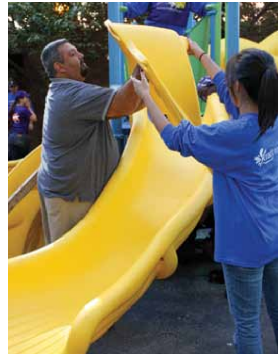
Playground equipment installed in one day.
